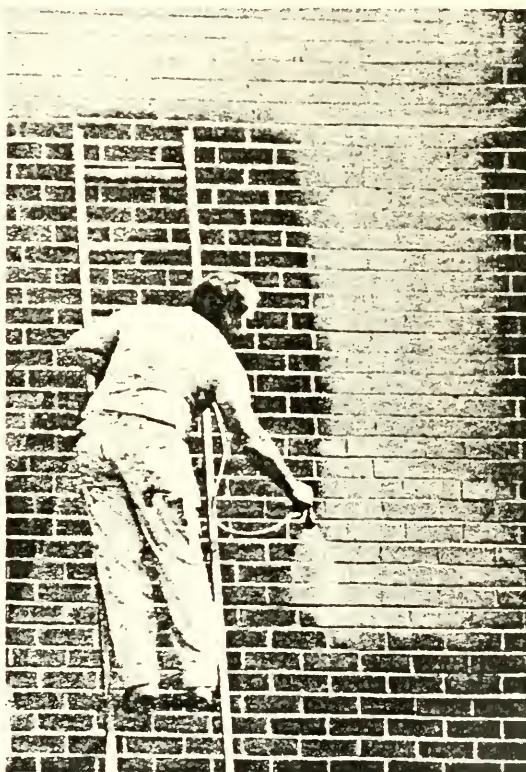
A construction worker at the Villages of Montpelier, formerly known as the Pumpkin Hill-South Laurel Apartments, sprays paint—not graffiti—on the brick wall of one of the buildings undergoing a complete overhaul at the complex east of the Baltimore-Washington Parkway and south of Route 197.
